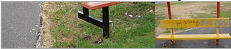
Goal Posts missing nets and cement bases lifted from ground
